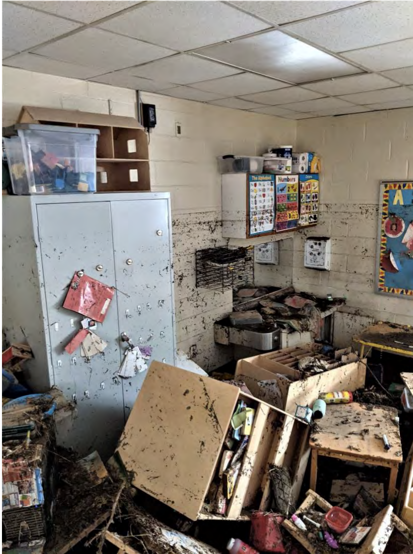
The walls in this prekindergarten room at Waverly Elementary School show that floodwaters rose higher than children's heads. (Vivian Spencer)
