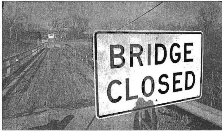
A wooden bridge that provided easy access into the subdivision was closed in September to become a footbridge. It spans the Glacial Drumlin Trail.
