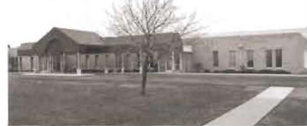
GOODWILL 21ST STREET FACILITY, RACINE, WIS.
